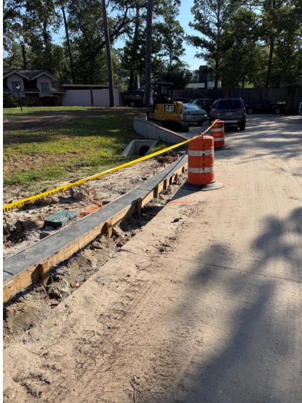
Figure 2: Ribbon Curb Looking East at end of Roadway
