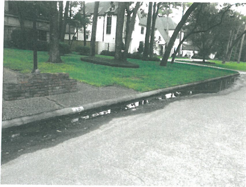
Location No. 20 – 19 & 23 Willowron Drive (1 of 2)
